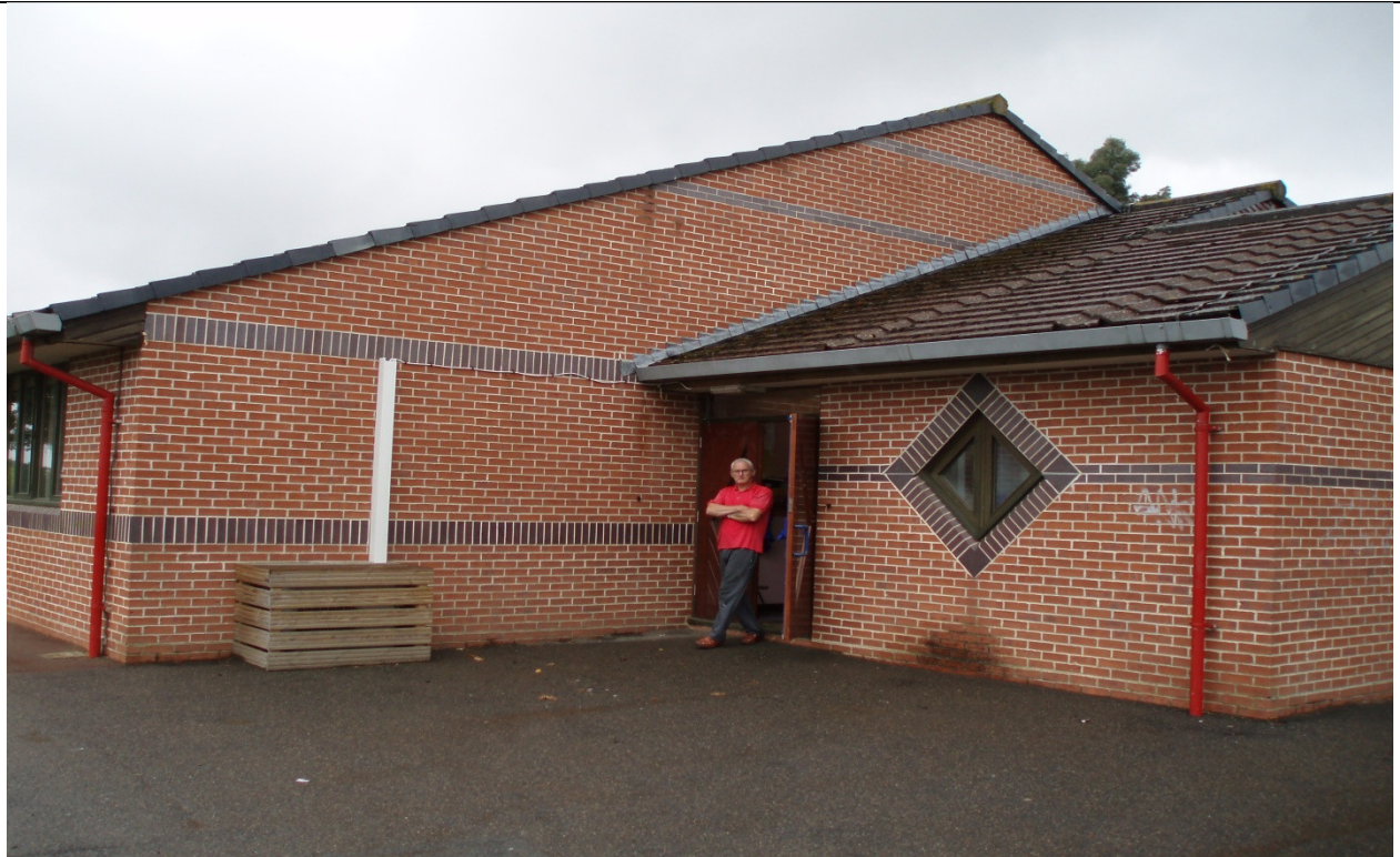
View of the existing area for the proposed extension, the projection of the flat roof to sit roughly along the line of the brick band from the end of the gutter line.
